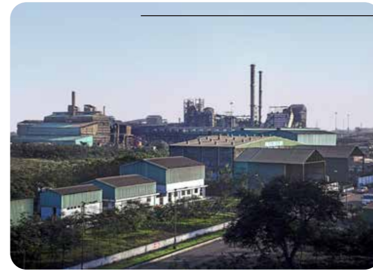
Pellet Plant Capacity 2.7 MTPA Utilisation levels: 90%
